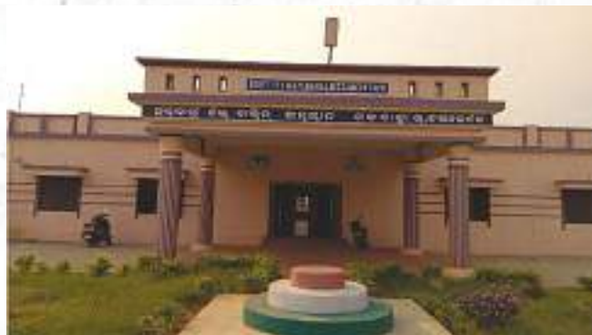
ITI Gajabahal, Odhisa constructed under LWE Scheme
