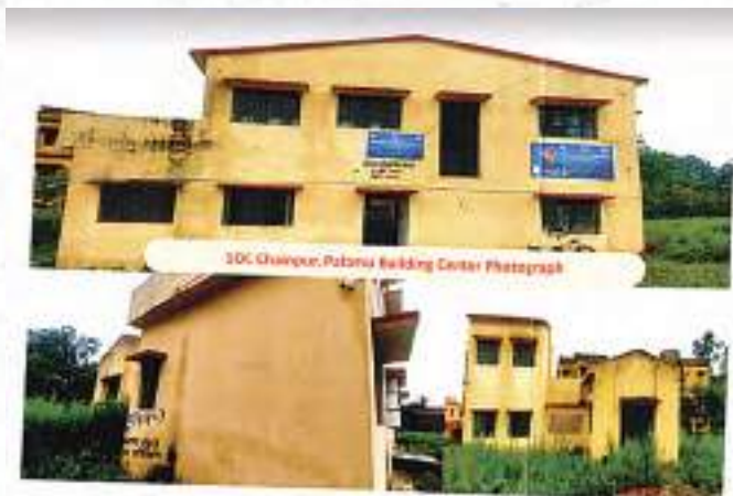
SDC Palamu, Jharkhand constructed under LWE Scheme
